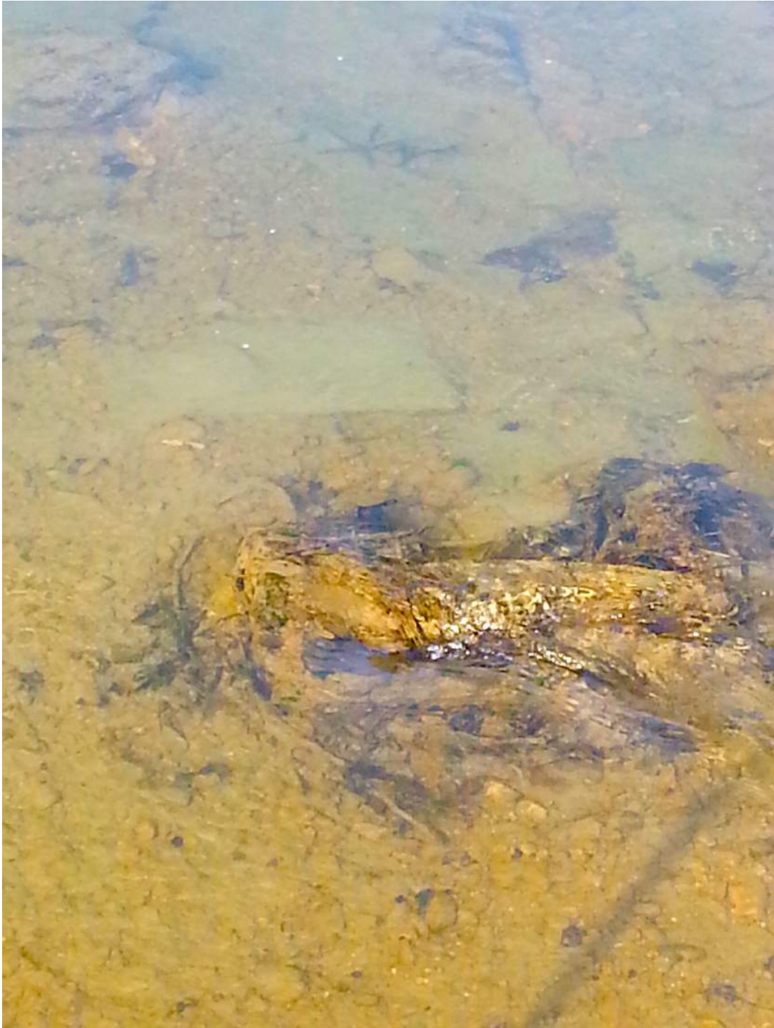
Triadelphia house stone floor slabs just upstream of foundation. Top half of image.
