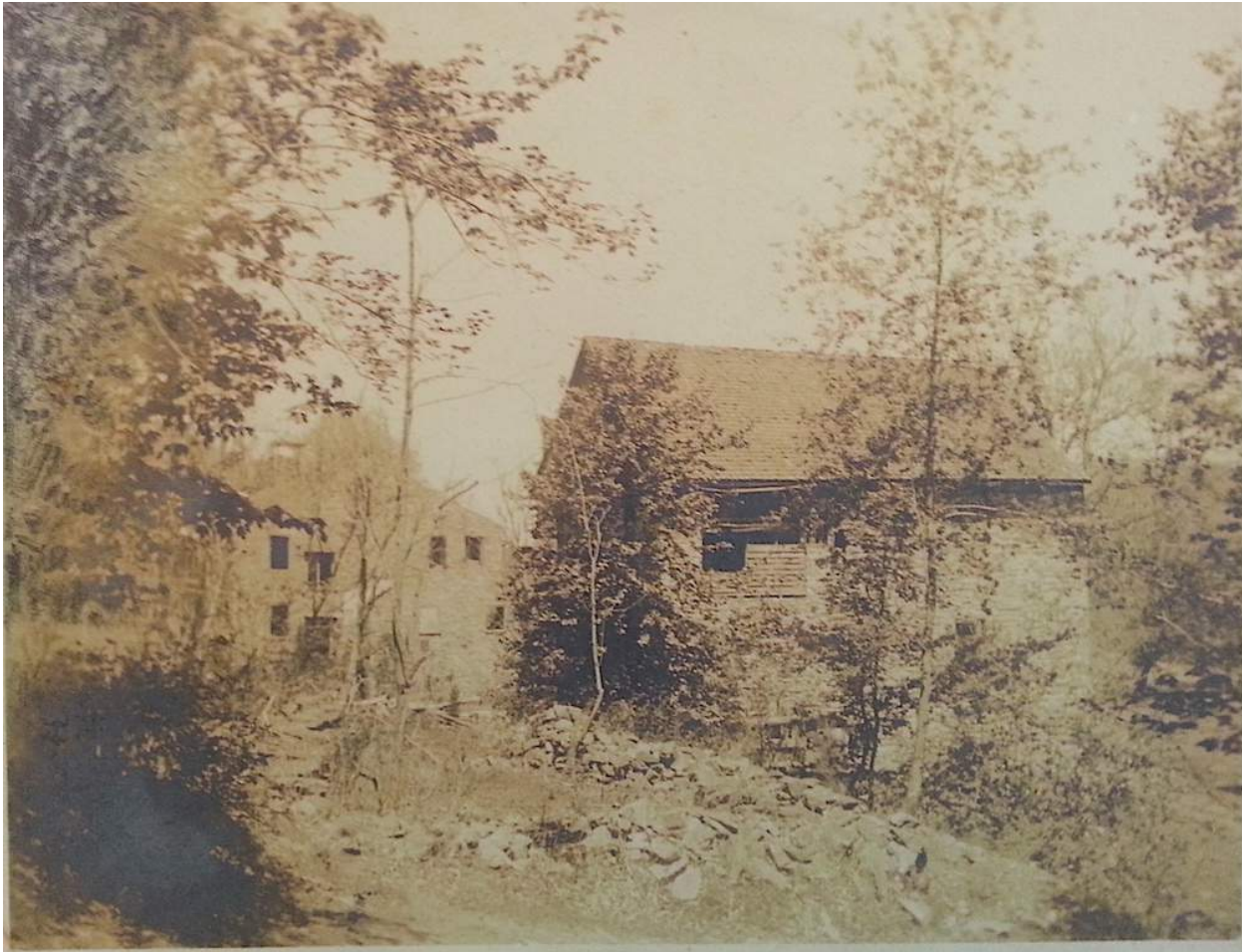
View of ruined foundation of Mill with south end of Cotton Factory seen to north. Mill appears to have been a frame structure on rubble foundation typical of many farm buildings of period. Proved not durable in the massive flooding of 1889 in which the massive stone buildings on
