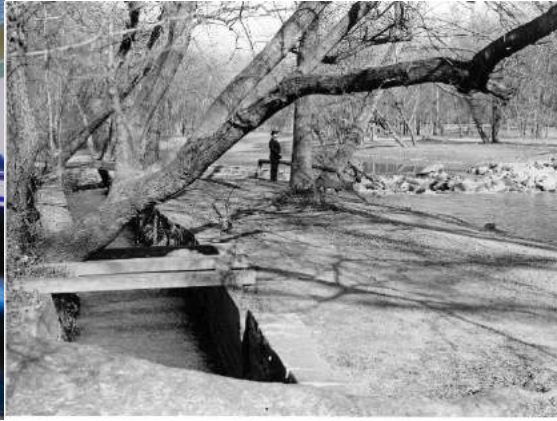
Mill stone layout and mill dam and head race of Isaac Peirce Mill in Rock Creek Park , Washington, D.C.
