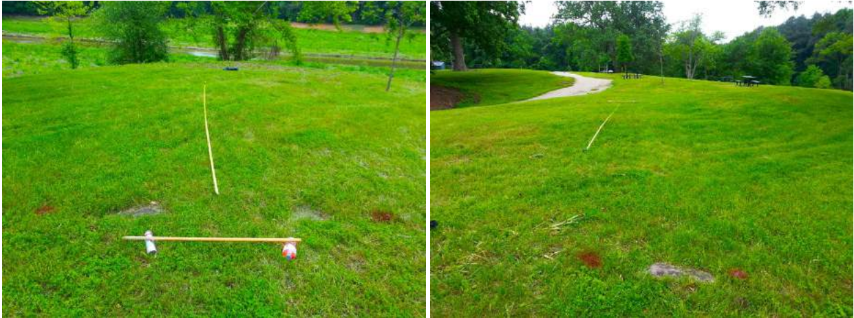
Exposed front (left) and rear (right) foundation stones. Church was 32' deep and 20' wide as determined from these stones and 1937 aerial photography.
