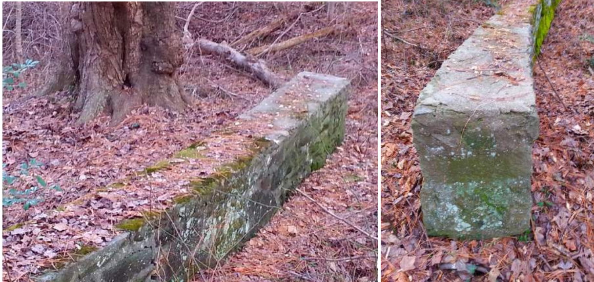
The Triadelphia Spring wall, an example of period stone work and wall thickness. Side and end.
