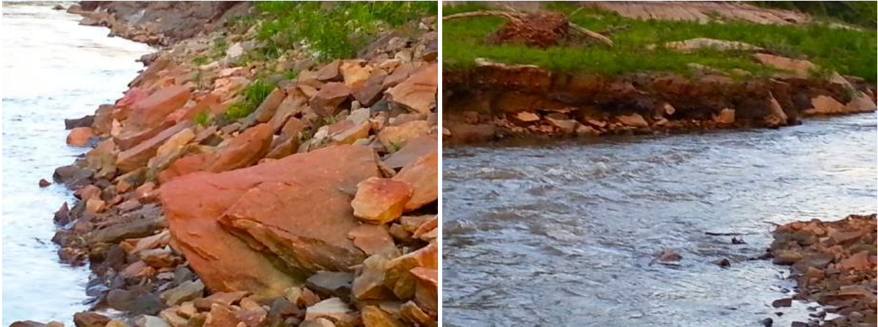
West and east bank foundation debris fields details
