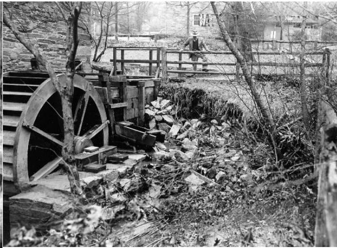
Pierce Mill head race detail showing uncommon stone facing, most were simply ditches and unrestored water wheel.
