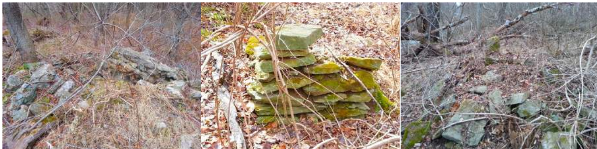
Examples of house ruins near Triadelphia: on back road past church site; overlooking Triadelphia from Howard County using flat stones like those used in dam face; on Triadelphia Lake Rd (old Triadelphia Rd) just above modern boat landing area. The first is cement but other two are dry, although period clay mortar may have been used.
