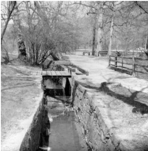
Pierce Mill head race detail showing uncommon stone facing, most were simply ditches and unrestored water wheel.
