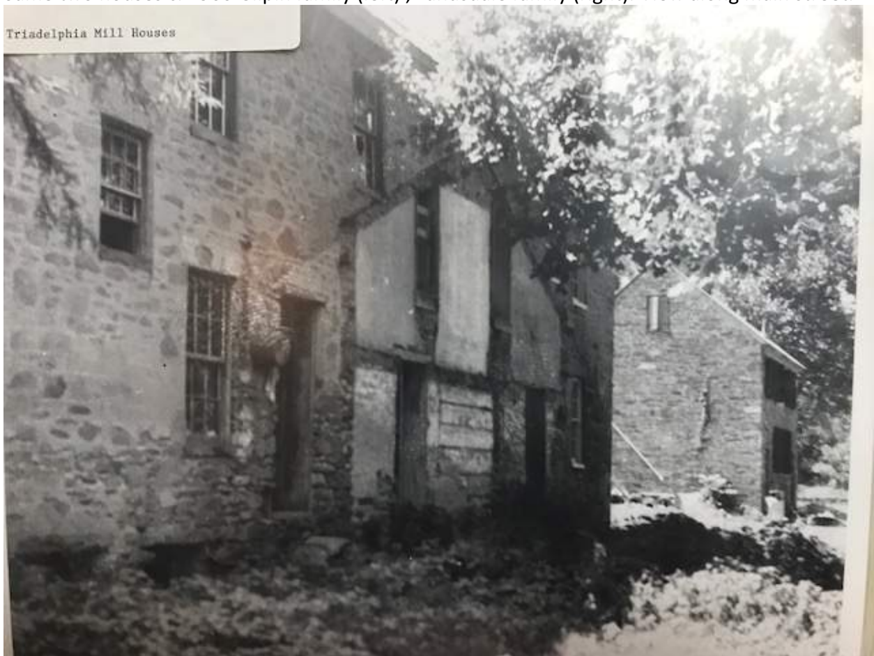
Backs of Lansdale house in foreground, Gilpin house background. Note trace of the removal of rear wing on Lansdale house. Trace indicates a frame structure with plastering that was done to
