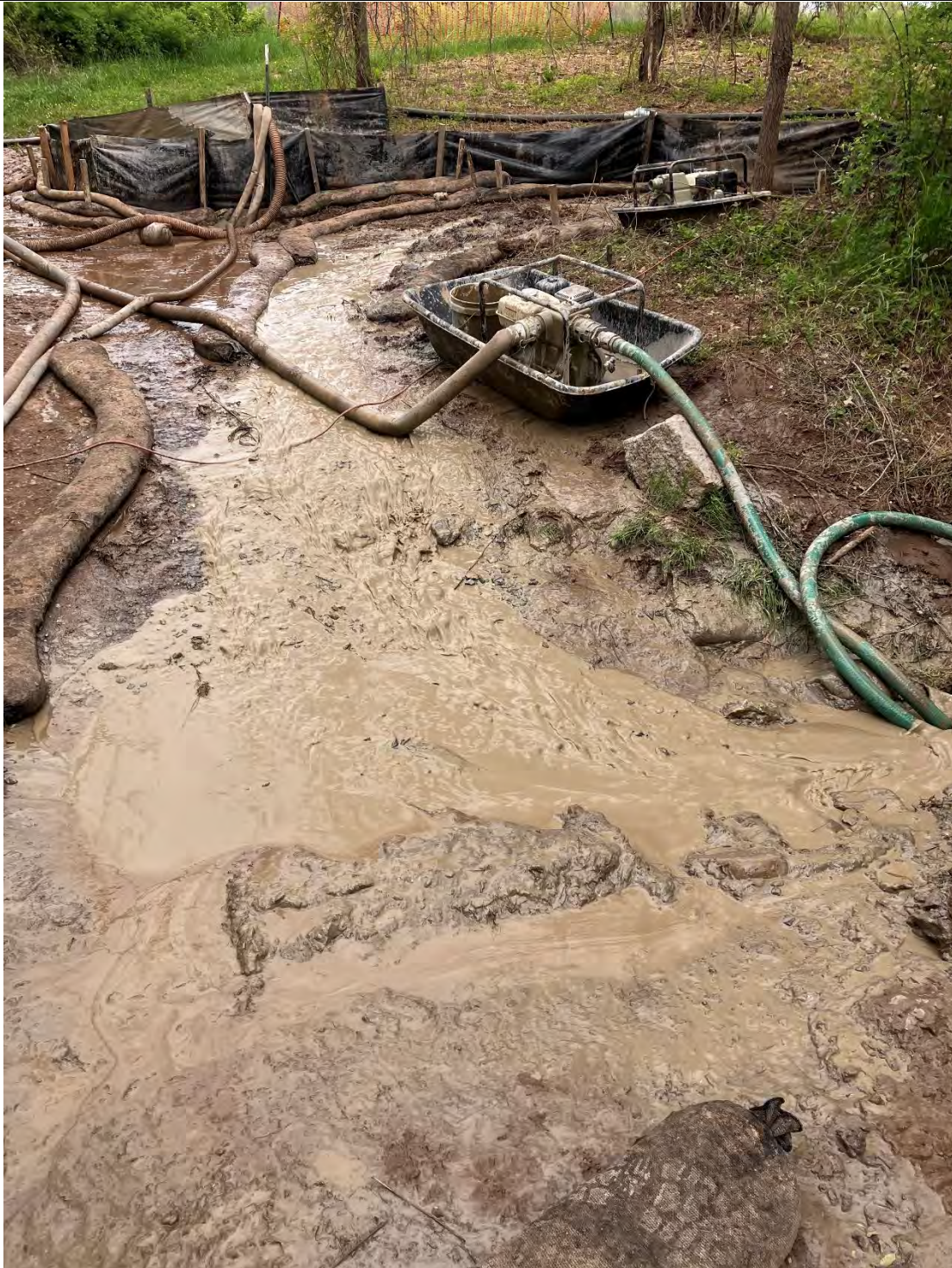
Figure E: The two frac-outs on the western bank of UT to Monocacy River are discharging into the waterway and are not individually contained. These frac-outs are located at Segment 2. The one frac-out is the same one documented in Figure A. Sediment (bentonite) pollution is occurring in the Waters of the State but is contained at a downstream point.
