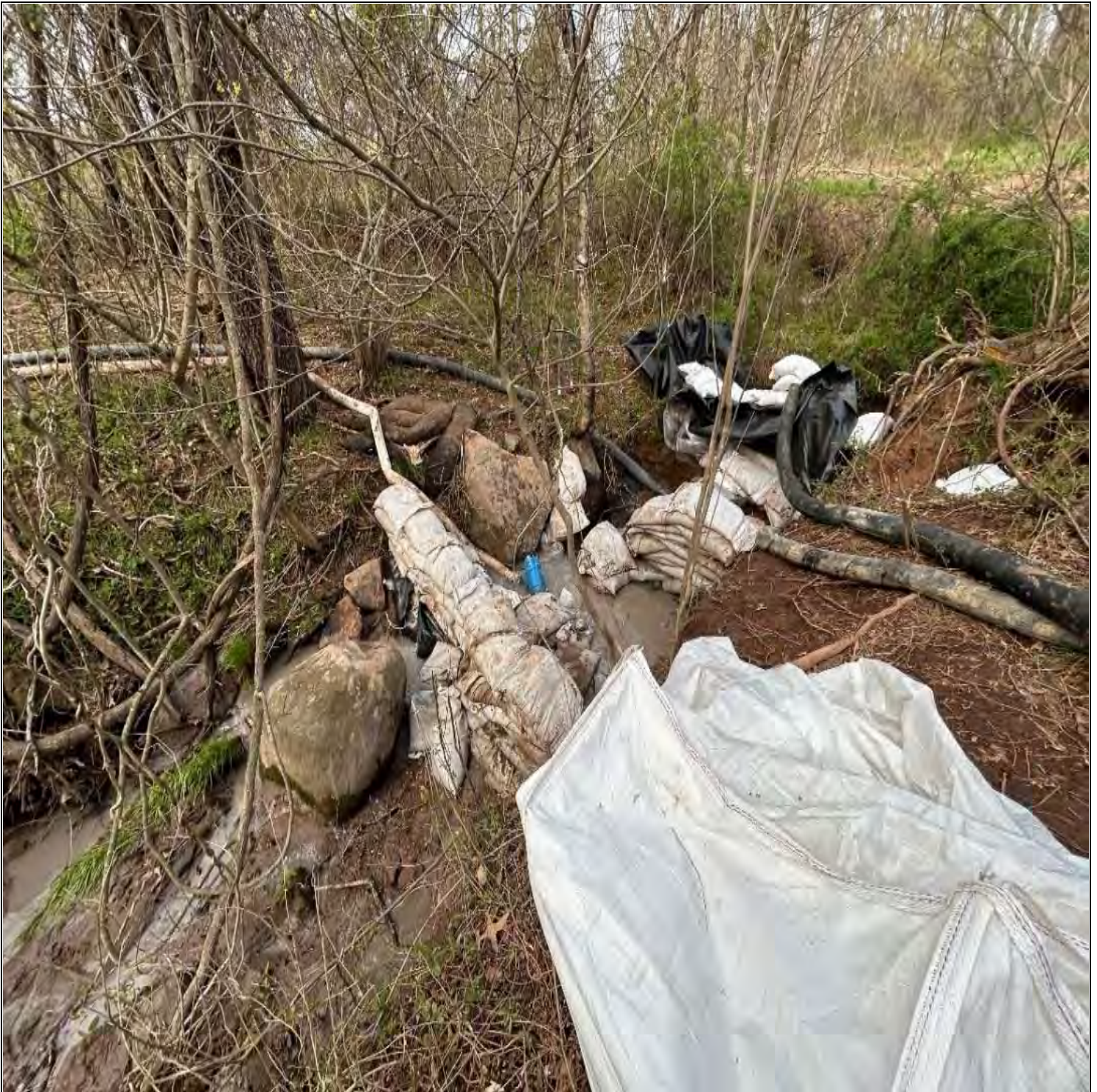
Figure H: "Origin/pumping area of tributary and the site of the bentonite discharge. Upstream is clearwater flow." The photo was taken on 04/08/2024 by Douglas Cochran with Frederick County Government.
