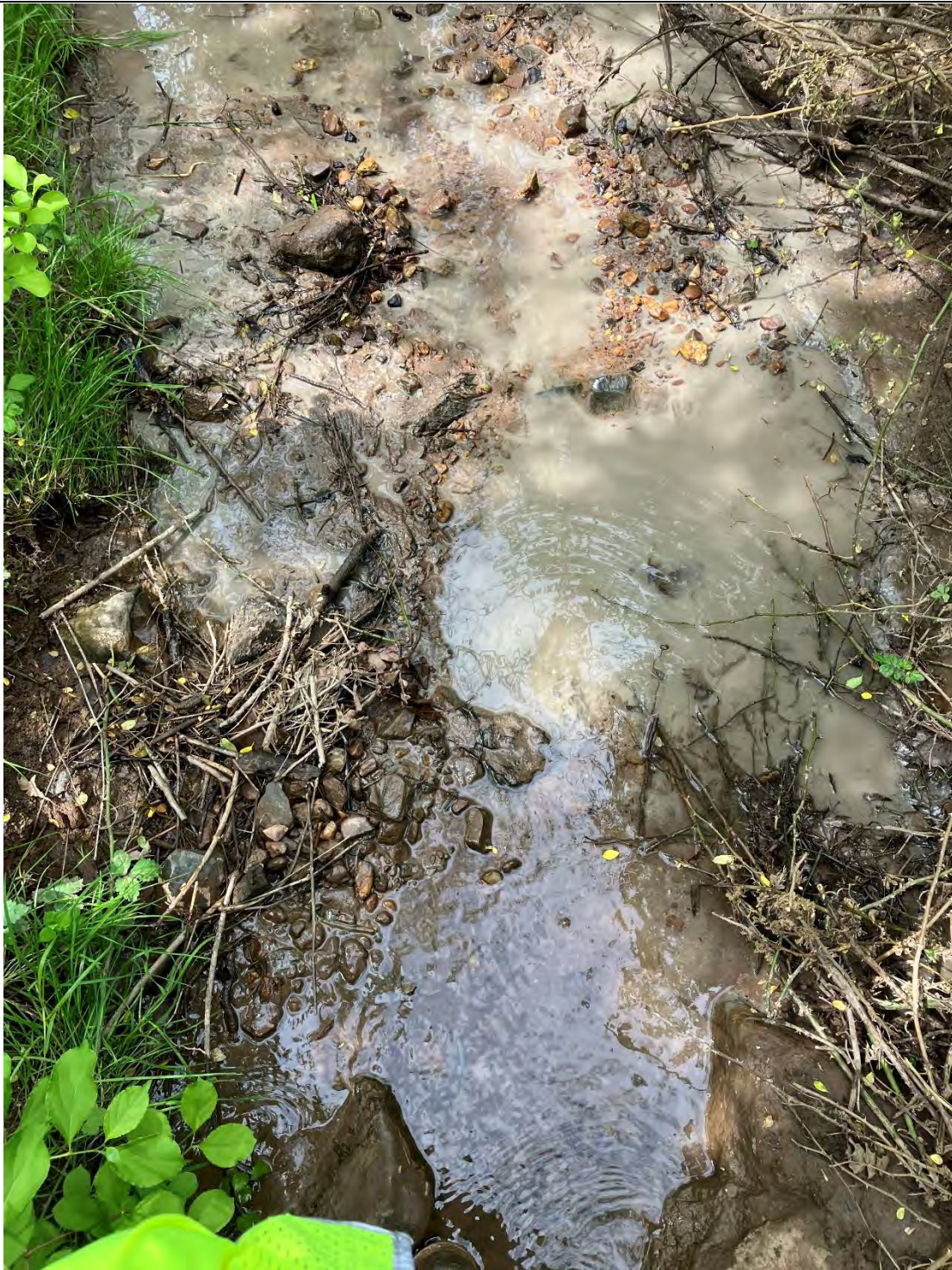
Figure C: The other undocumented frac-out was within the stream (UT to Monocacy River, use class I-P waters) channel just downstream of the documented (in the 04/10/2024 MDE inspection report) frac-out (frac-out in Figure B) that was contained with sandbags around the discharge point. This frac-out is located at Segment 2. Sediment (bentonite) pollution is occurring in the Waters of the State but is contained at a downstream point.
