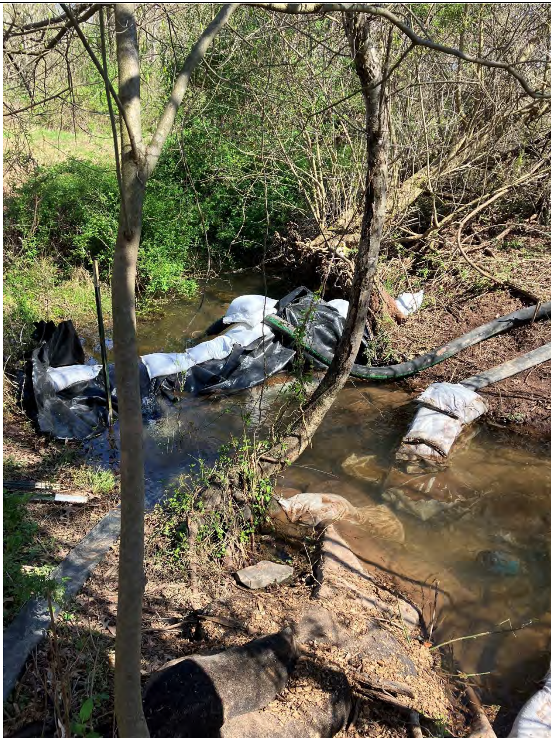
Figure D: Another frac-out was within the channel of a waterway (UT to Monocacy River, use class I-P waters), and the discharge point was located underwater on the stream bank. All of the frac-outs that occurred in the waterway (UT to Monocacy River, use class I-P waters) had sandbag containments around the discharge points; the containment was utilized to help to isolate and pump out the sediment-laden discharge water. Sediment (bentonite) pollution was found in the Waters of the State and remains in a condition likely to continue to pollute.
