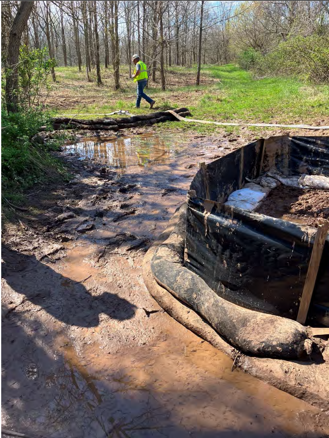
Figure F: Outside of the frac-out documented in Figure E there was sediment (bentonite) deposition. Sediment pollution was found in the Waters of the State and remains in a condition likely to continue to pollute. There was substantial sediment (bentonite) pollution downstream of where the frac-outs were located.
