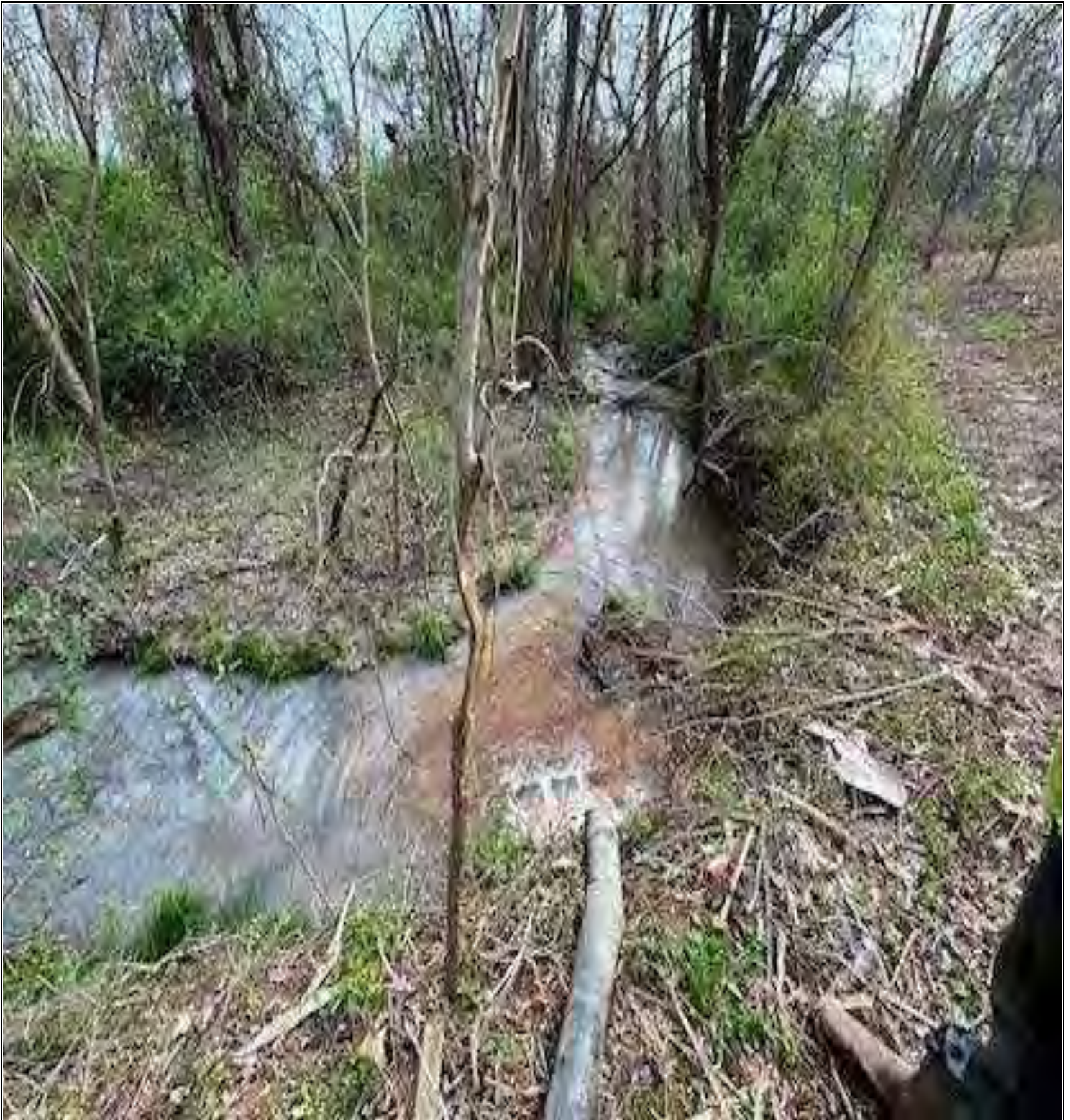
Figure L: "Clearwater pump around discharge to turbid streamflow downstream of containment area." The photo was taken on 04/08/2024 by Douglas Cochran with Frederick County Government.
