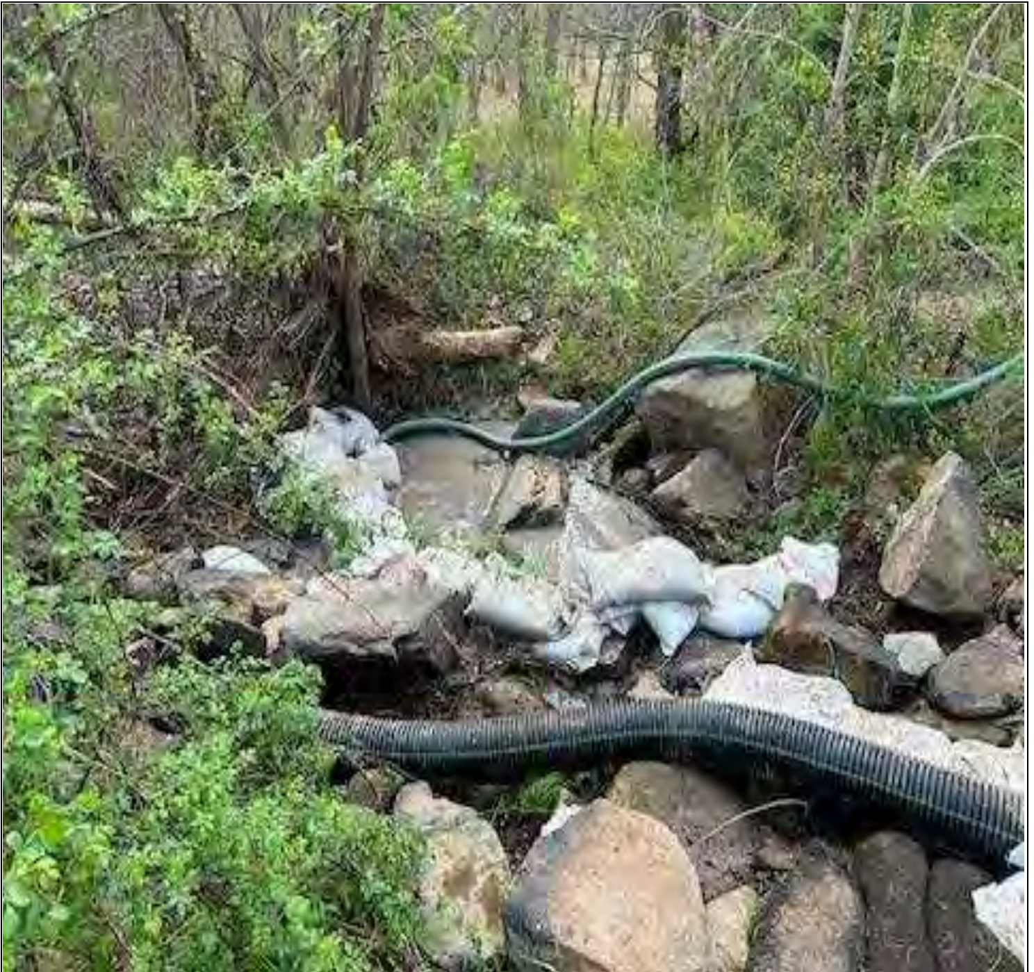
Figure 1: "Bentonite mud and drilling fluid present further downstream." The photo was taken on 04/08/2024 by Douglas Cochran with Frederick County Government.
