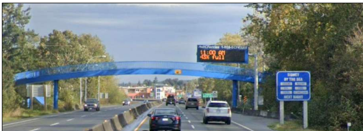
Figure 4-20: Variable Message Sign on Highway Approach to Sidney-Tsawwassen Ferry in Victoria, Canada
