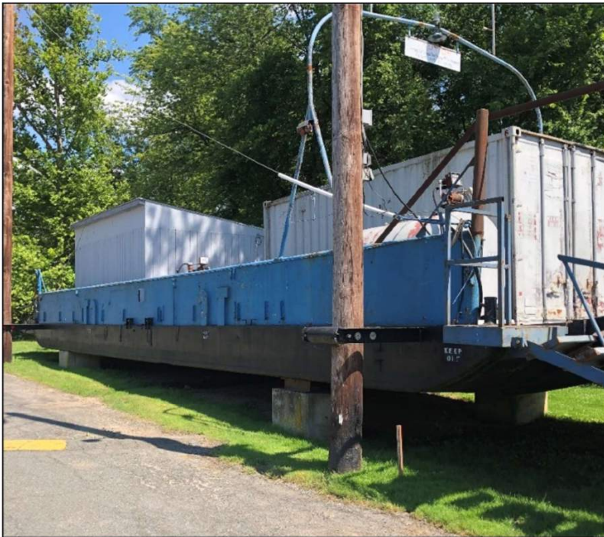
Figure 3-19: Old Ferry Barge Used for Fuel Storage Secured with Float Rails to Accommodate River Flooding
