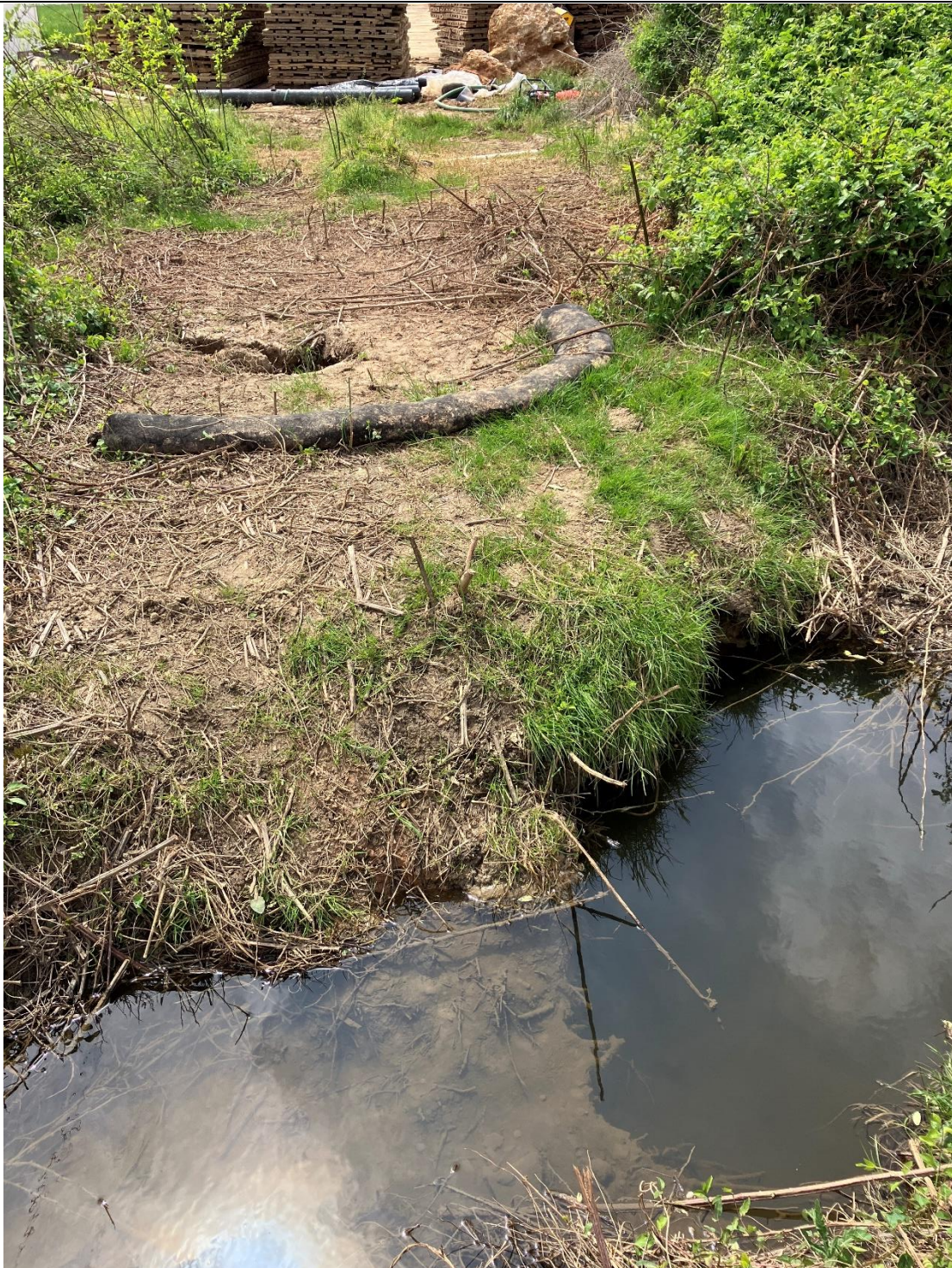
Figure G: There were cracks/fractures in the ground, noticed at the frac-out location in Segment 16 (located at roughly 39.3158900, -77.4996900). This frac-out has been cleaned up but the cracks/fractures have not been stabilized. Sediment (bentonite) pollution has occurred in the Waters of the State but was contained during the time of the inspection.
