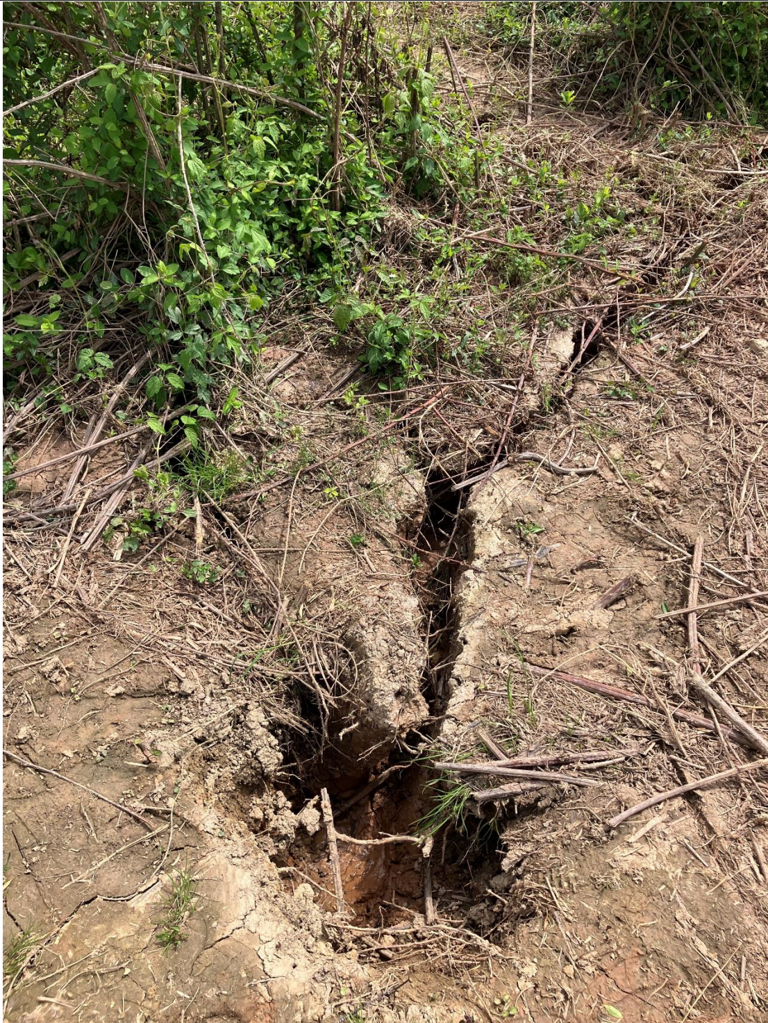
Figure F: There were cracks/fractures in the ground, noticed at the frac-out location in Segment 16 (located at roughly 39.3158900, -77.4996900). Sediment (bentonite) pollution has occurred in the Waters of the State but was contained during the time of the inspection.
