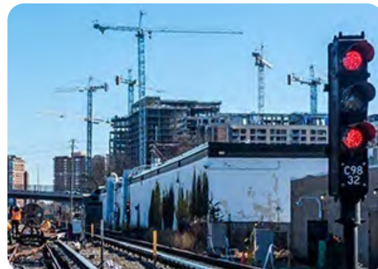
Next-Gen Automation and Signaling
