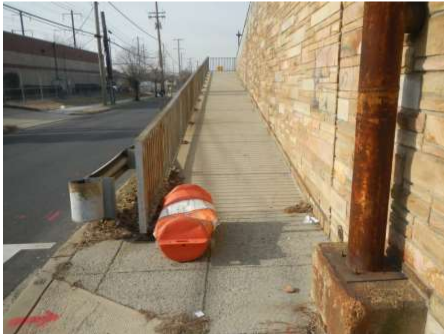
Photograph No. 6 – Lower Southeast Approach Pedestrian Ramp (Looking South)
