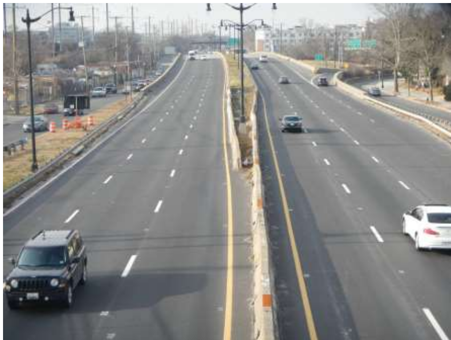
Photograph No. 10 – Looking South From Top of Bridge at Mid-Span
