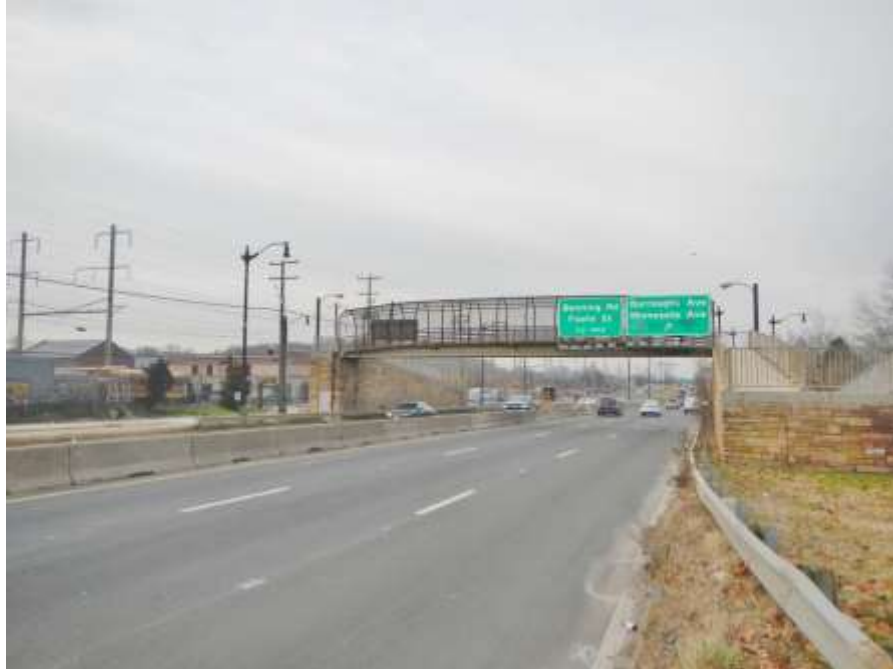
Photograph No. 1 – North Elevation (Looking Southeast)
