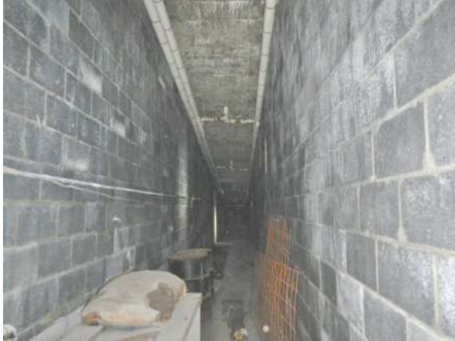
Photograph No. 37 – View Inside West Abutment Under Upper Pedestrian Approach Ramp
