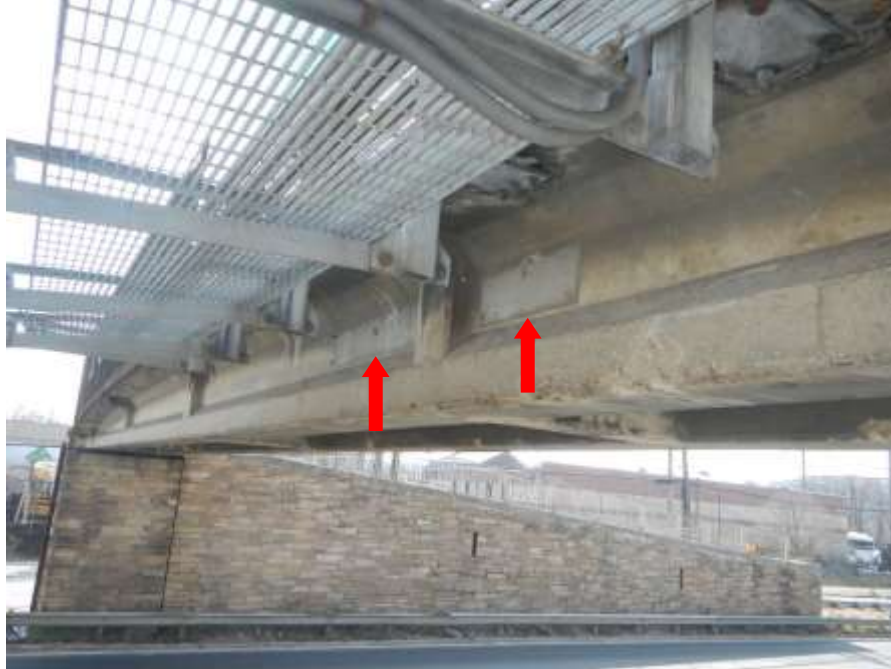
Photograph No. 49 – Both Sections of "Clearance 14 Ft." Sign Missing Above Southbound Lanes (Looking Southeast)
