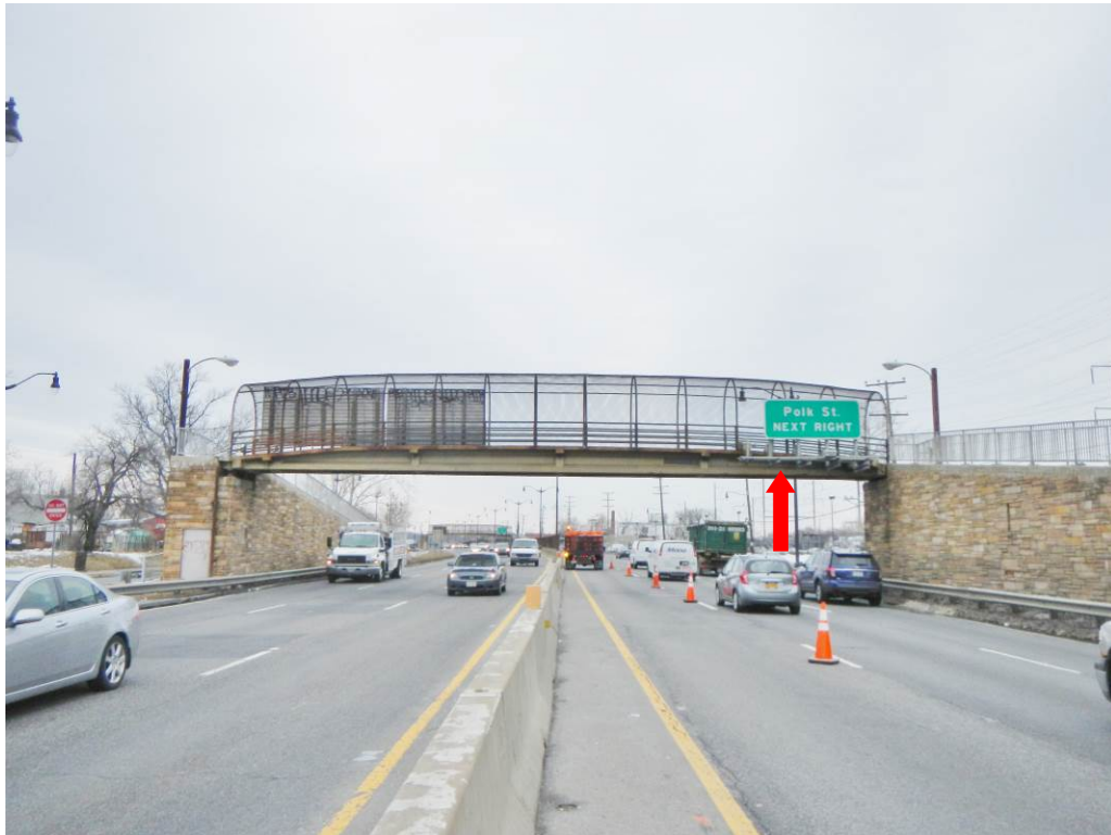
Photograph No. 1 – South Elevation (Looking North): Showing Location of Delaminated and Loose Concrete
