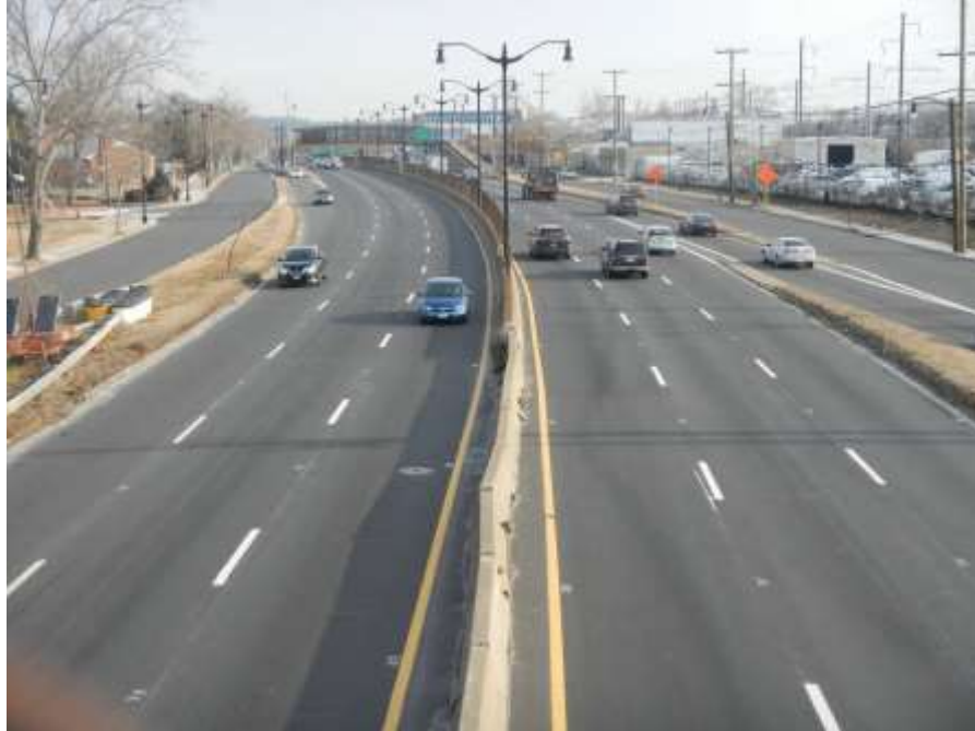
Photograph No. 9 – Looking North From Top of Bridge at Mid-Span
