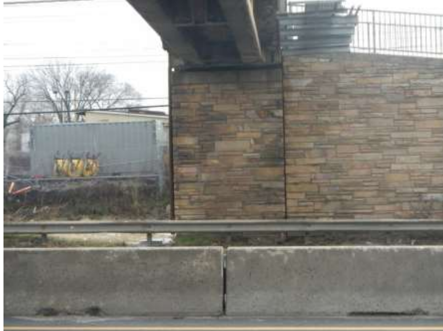
Photograph No. 33 – East Abutment Elevation
