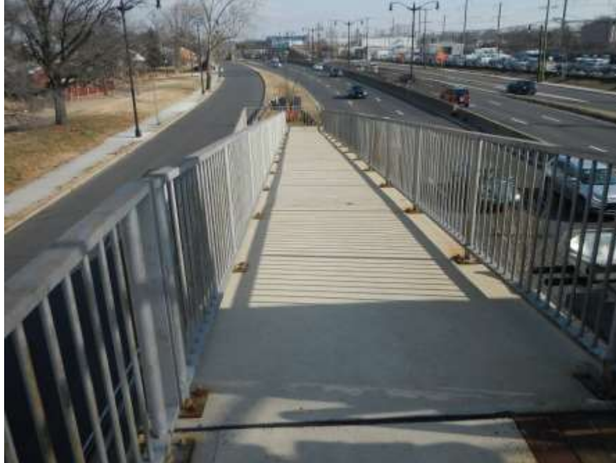
Photograph No. 5 – Upper Northwest Approach Pedestrian Ramp (Looking North)
