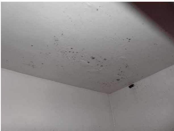
Visible mold growth on bathroom ceiling
