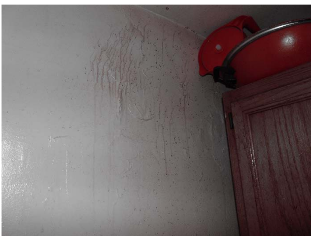
Visible mold growth and water damage to kitchen walls
