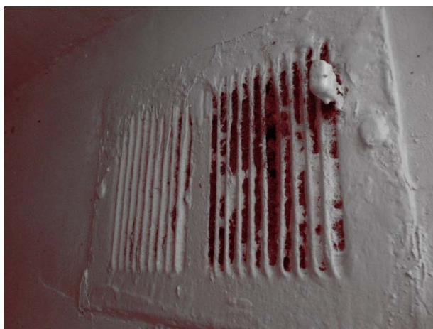
Bathroom vent completely clogged
