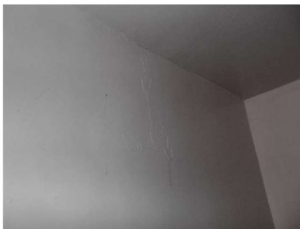
Water damaged living room ceiling (adjoining impacted kitchen wall)
