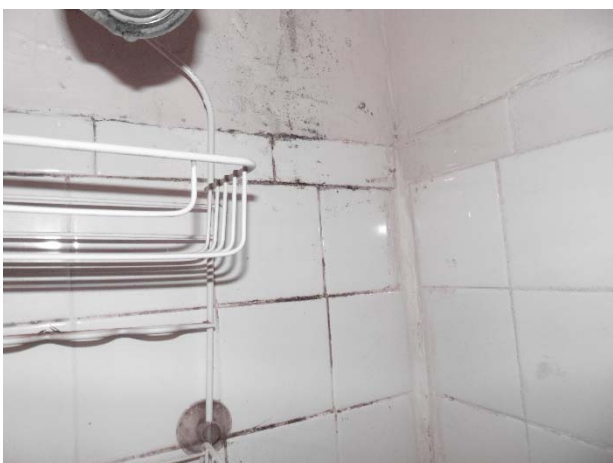
Mold growth on bathroom walls
