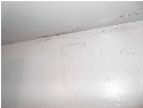
Mold growth on bathroom ceiling and walls
